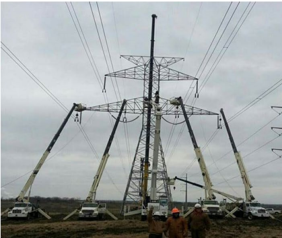
Traditional Lifting Method (costly cranes and heavy footprint)
