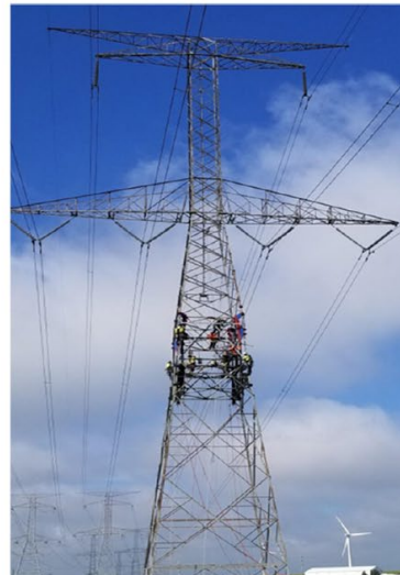
AMPJACK® Raise Method (no cranes and minimal footprint)
